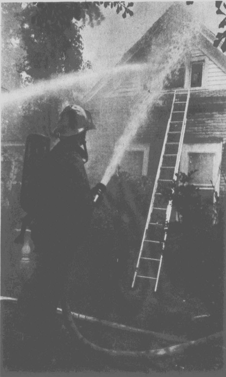
EARLY MORNING FIRE — A fireman sprays water on a house at 701 W. Fourth Street early today when a fire started there in the attic. According to Greenville Fire Chief Jenness Allen, a woman and two children were in the house but were gotten out by a building inspector who was passing by. No one was injured in the fire. (Reflector Photo by Cliff Hollis)
