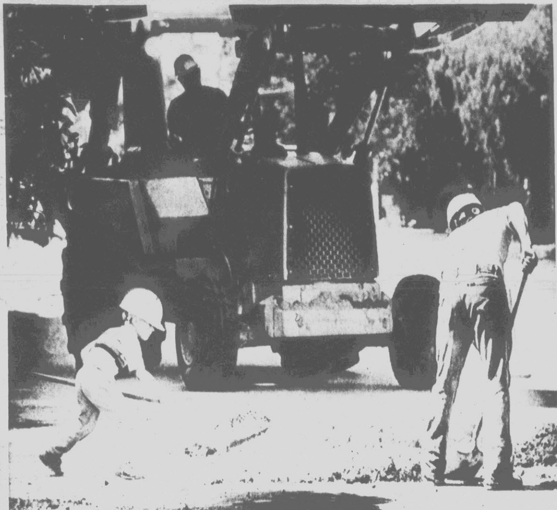
A LITTLE HELP — Five-year-old Eddy Klier of San Carlos, Calif., mans the broom to help his father and other members of a construction company install a water main. The joint effort came on a repair project on a residential street in Atherton, Calif. (AP Laserphoto)
