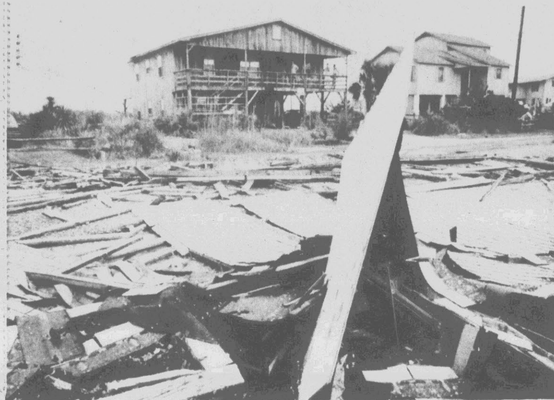
S.C. DAMAGE — Occupants of a beach house stand on the porch, background, while looking at a section of the roof which was blown from their house in Garden City, S.C., Wednesday afternoon during a severe
