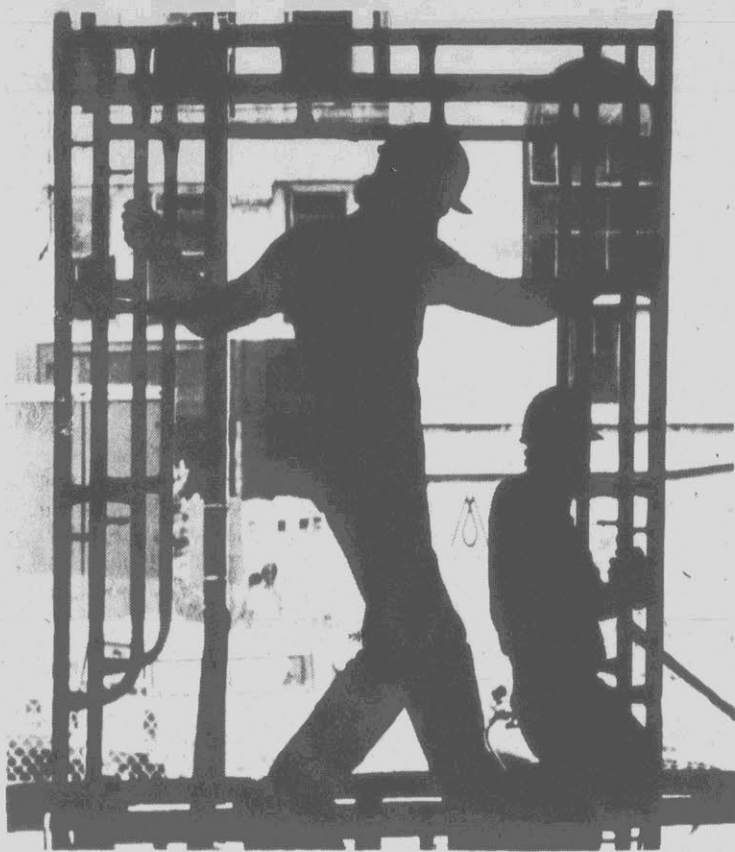
SCAFFOLD ARTISTRY — Construction workers Mike Nix and Michael Byrum erect scaffolding inside a building in downtown Asheville, creating an artistic styling as they make preparations for more work. The building is being gutted for renovation as part of Asheville's downtown revitalization project. (AP Laserphoto)
