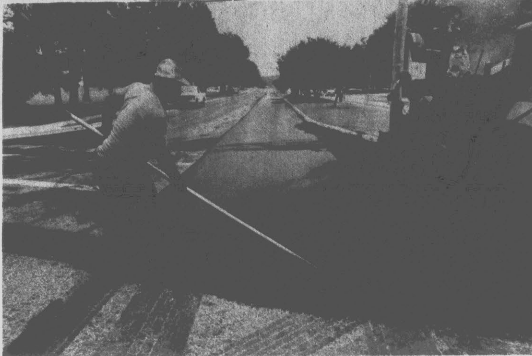
RESURFACING STREET — Workman Timmy Barnes smooths new asphalt at the intersection of 14th and Elm streets Monday, part of a repaving project for Elm. According to Glenn Whistler, assistant city
