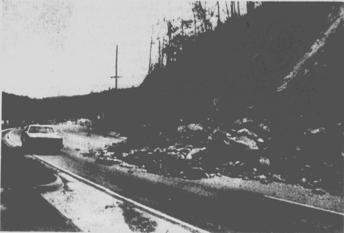
DETOUR — Law enforcement officials set up detours from a segment of U.S. 321 near Boone late Saturday in anticipation of a rock slide that eventually occurred Sunday afternoon. Traffic between Boone and Blowing Rock is now being diverted to the Blue Ridge Parkway. (AP Laserphoto)
