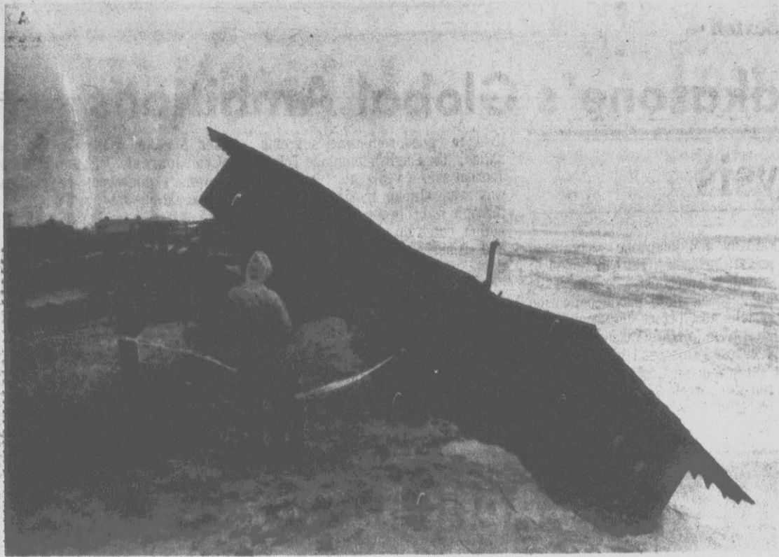
DESTROYED HOUSE — This one-story, four-bedroom vacation house was destroyed Sunday by the pounding surf at Nags Head. The house, which earlier had been condemned because of erosion under its pilings, fell off the foundation posts Sunday and slid down the steep dune toward the beach. (AP Laserphoto)
