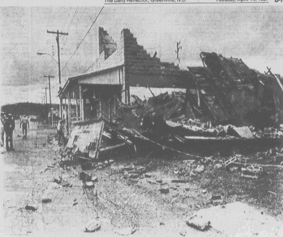
STORM DAMAGE — Tornado winds leveled this store building and 20 other structures in Branch, Ark., on Monday. A tornado also peeled off the roof of an elementary school in Bergman, Ark., and struck a mobile home park in Green Forest, Ark. Four people were injured, authorities said. (AP Laserphoto)
