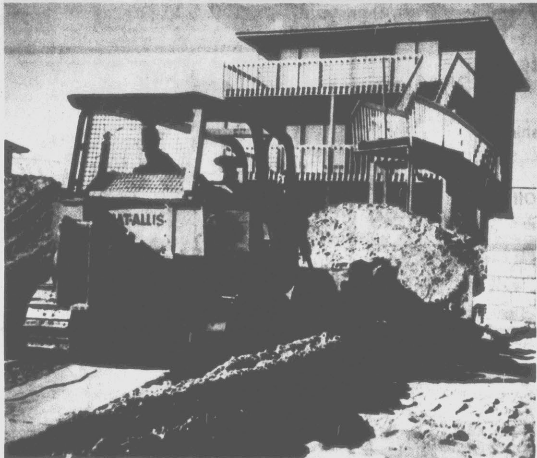
DUNE WORK — A bulldozer reconstructs dunes lost during storms earlier this winter at Topsail Beach. The town is on the southern end of Topsail Island, where development has become a controversial topic. (AP Laser-photo)
