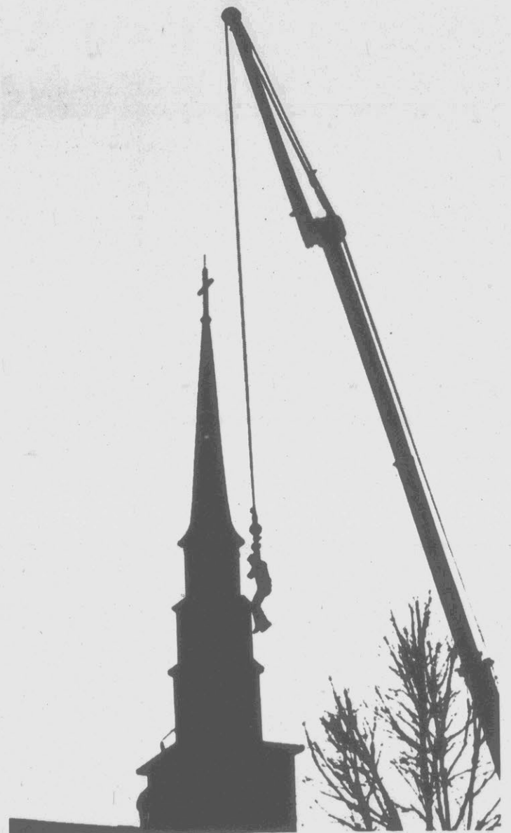
SWINGING IN THE BREEZE — Workers place a 47-foot steeple in place on the Landis Baptist Church in Landis. The workman hanging on the end of the crane cable, Rodney Caudle, was disconnecting the lines used to lift the top of the steeple into place. Installed, the top of the steeple rose 90 feet above the ground. (AP Laserphoto)
