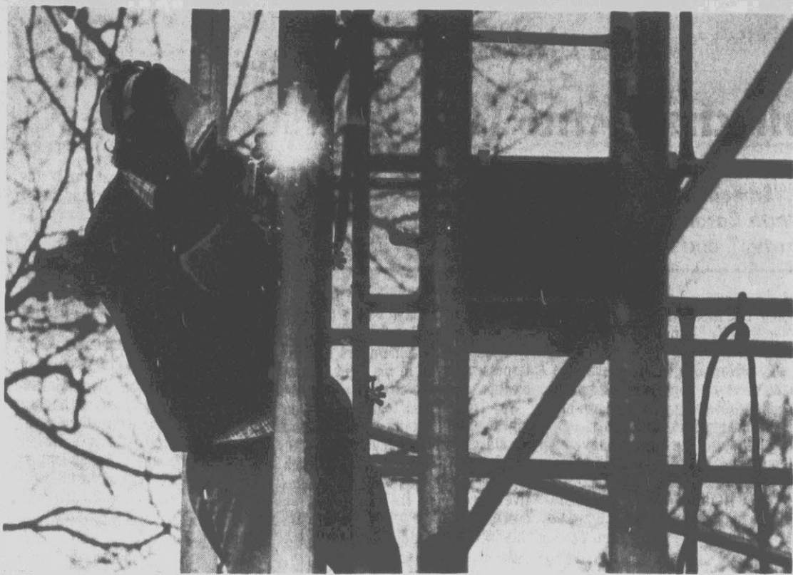
WAY UP THERE — Euerardo Machado went to great heights to do his job in Elm Street Park Wednesday afternoon. He was part of a crew of workers putting up a backstop on the park's baseball diamond. Machado's responsibility was to weld — way up high on the scaffolding. (Reflector Photo by Cliff Hollis)
