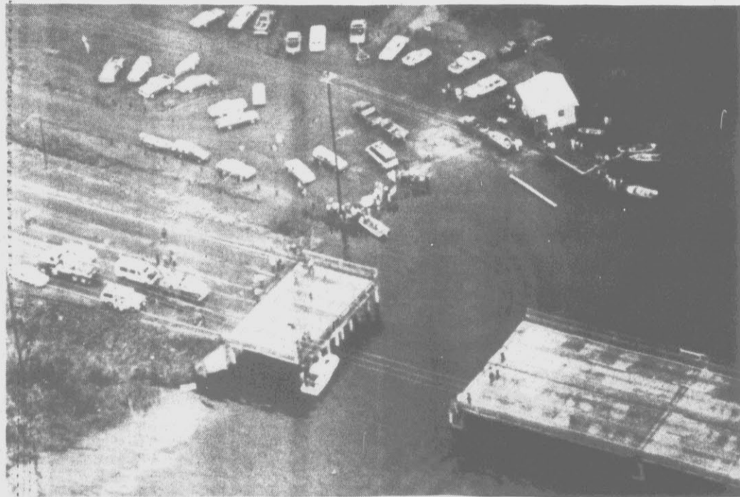
TRANSPORTATION GAP — A section of the U.S. 43 bridge over Chickasaw Creek near Mobile, Ala., collapsed Wednesday, leaving a 68-foot section open as a greeting for commuters this morning. Rescuers used
