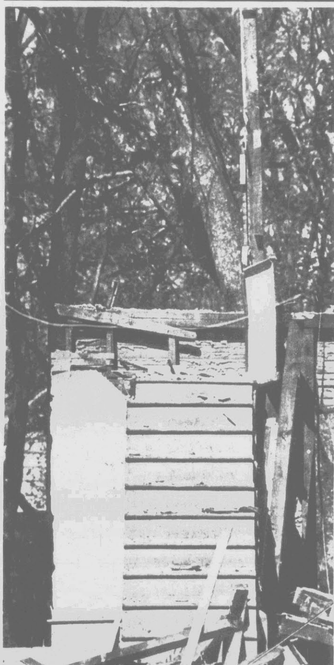
STAIRS TO THE TREES? — What appears to be stairs to the trees is really a staircase left during the demolition of an old house on Evans Street recently. Workers demolished the house, leaving the steps for last. (Reflector Photo by Tommy Forrest)
