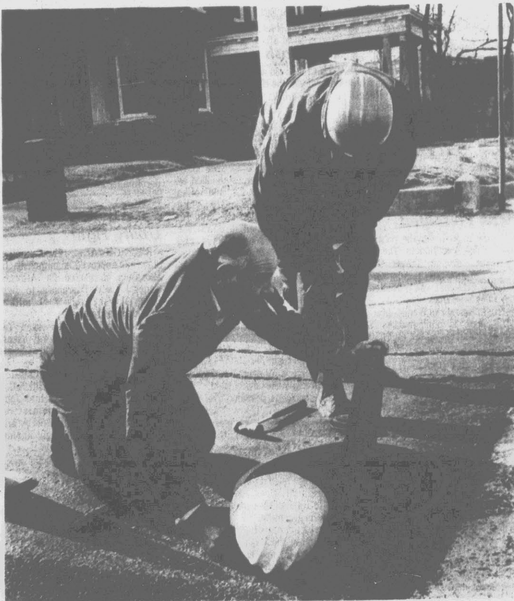
CHECKING THE LINES — George Mayo and Joseph Shelley check a manhole on Cotanche Street in preparation for installing new gas lines. Greenville Utilities work crews will install a line from Cotanche Street to Holly Street as part of an ongoing effort to improve gas service throughout the city. (Reflector Photo by Chris Bennett)
