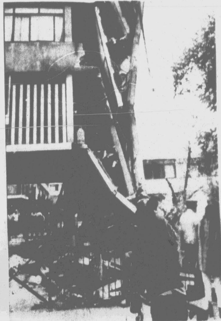
COLLAPSED BUILDING — One wing of a modern apartment building in Santiago, Chile, collapsed during a massive earthquake that struck much of central Chile Sunday. Authorities said 124 people were killed and 2,000 were injured in the earthquake. (AP Laserphoto)
