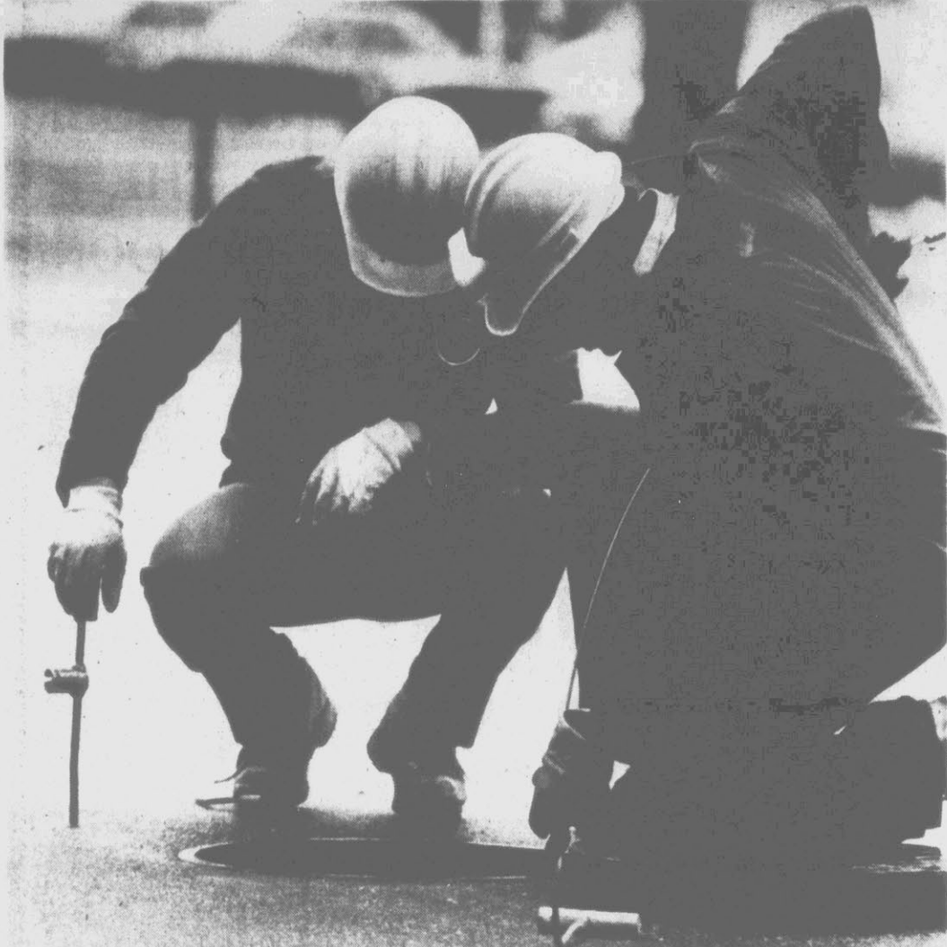
CLEANING JOB — Greenville Utility workers from the Water and Sewer Department, Ronnie Cox, left, and Ronald Smith give a sewer line on 8th Street a good cleaning as part of the city's normal maintenance routine. Drainage lines have had a workout in recent weeks with snow, rain and the ensuing debris putting a heavier-than-normal chore on them. (Reflector Photo by Tommy Forrest)
