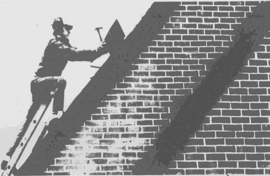
NAILING IT DOWN — Augusta, Ga., roofer Jeff Meeks stretches to put a shingle in place on the roof of Bethlehem Advent Christian Church. Meeks is part of a crew putting a new roof on the facility. (AP Laserphoto)
