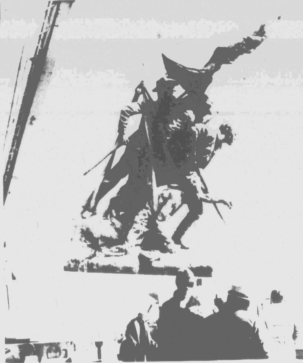
RESTORATION — North Carolina's monument at the Civil War battlefield in Gettysburg, Pa., is lifted on to a truck for shipment to a restoration plant in Cincinnati Wednesday. The monument, showing five soldiers
