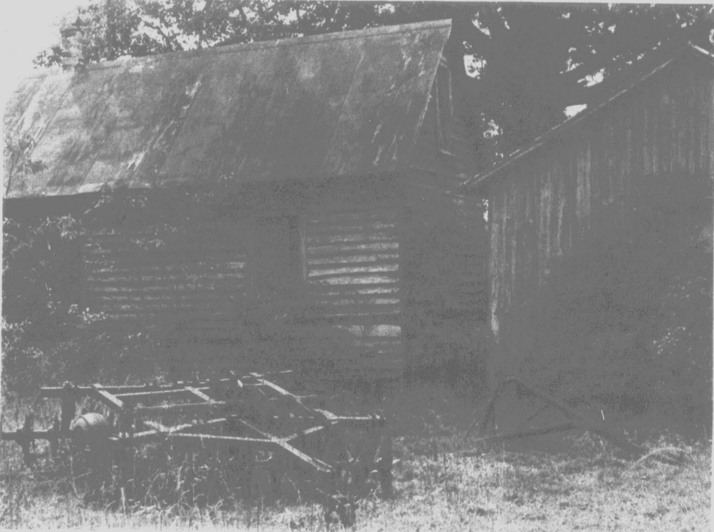
... The back view of the main house, left, and the detached kitchen, right, shows the narrow open passageway, called a breezeway, that separate the two structures. The breezeway separation
