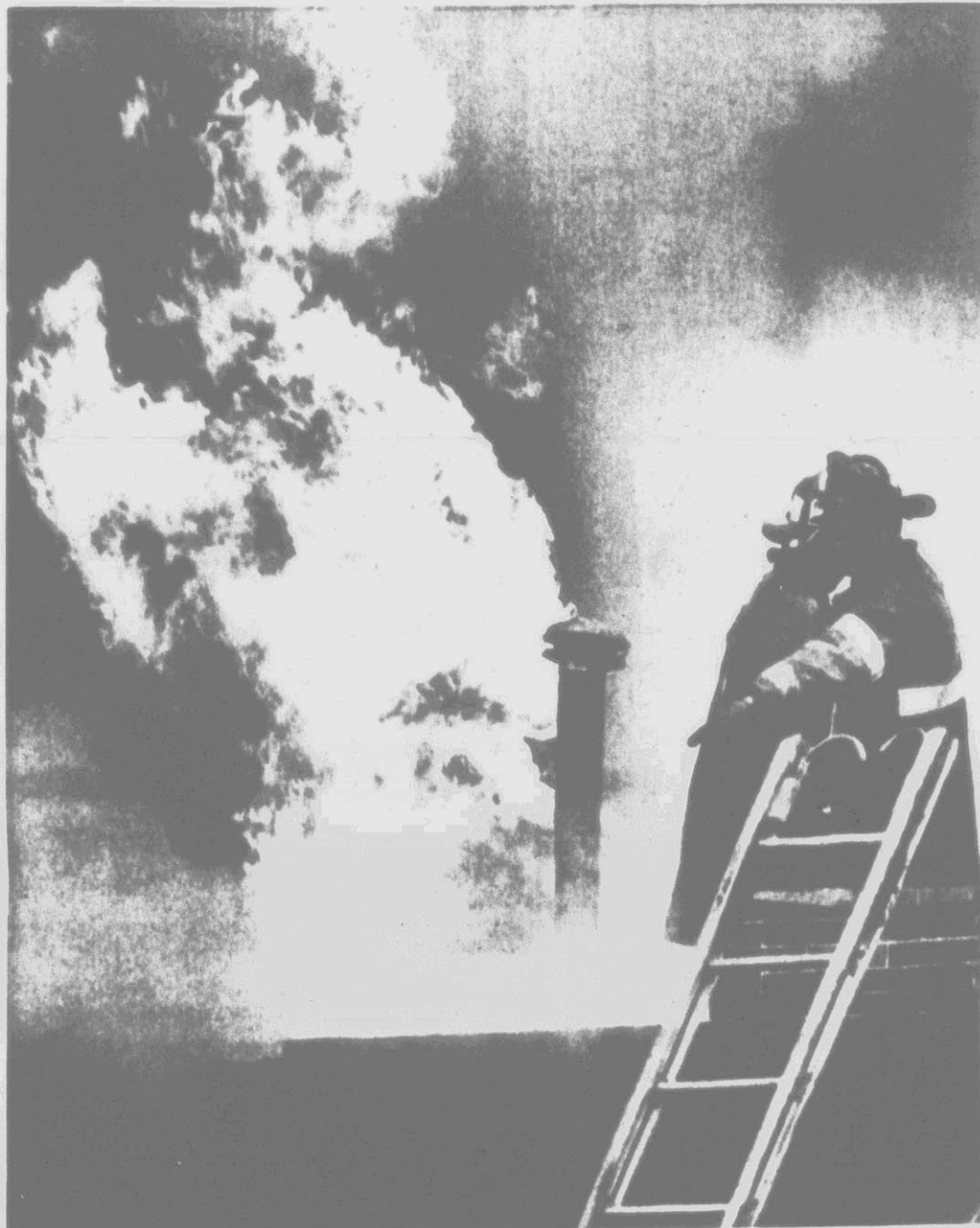
BALL OF FIRE — A firefighter points toward ground personnel today as a ball of fire shoots from the roof of a century-old market building in Boston's Haymarket
