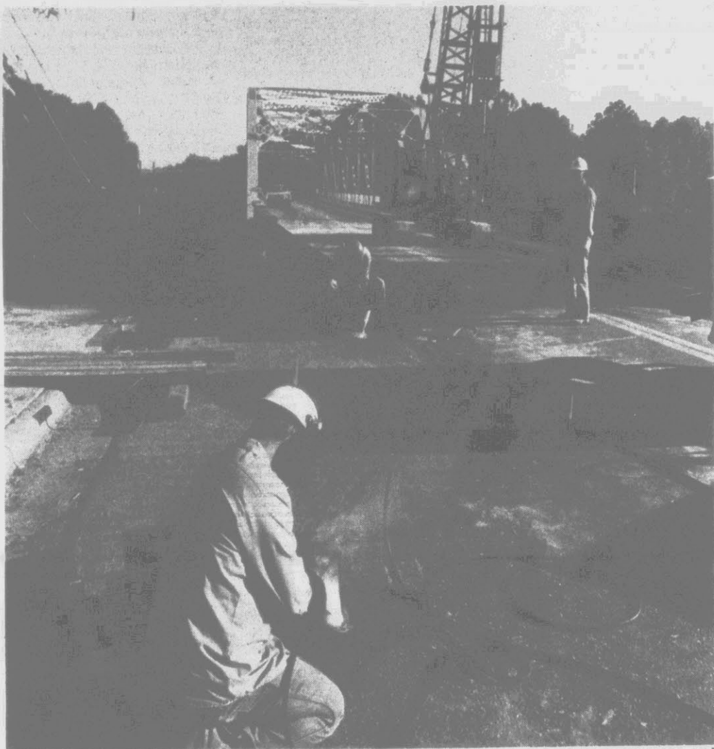
BRIDGE WORK — State Department of Transportation crewmen give the Greene Street Bridge a facelift in a periodic preventive maintenance project. DOT spokesmen say a new girder support cap and pilings should be in place by Thursday. (Reflector Photo by Tommy Forrest)
