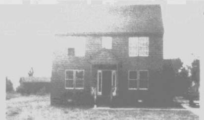
Pollard Construction Co. 102 Joseph Place Cherry Oaks
