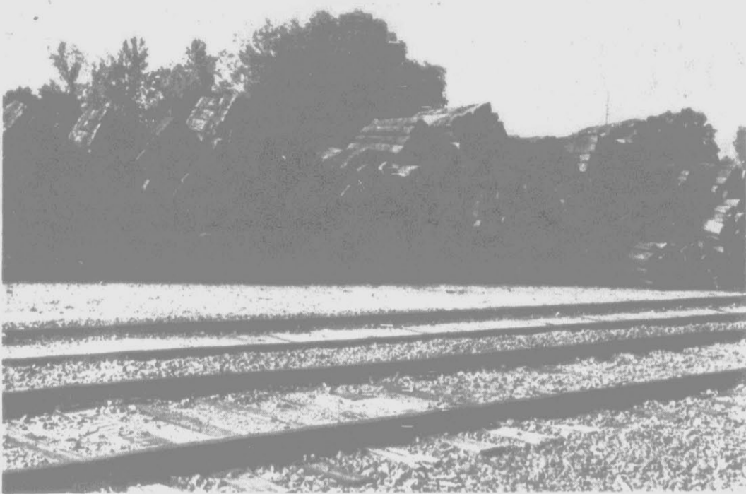
SALVAGE OPERATION — A long row of railroad ties are stacked along tracks off 14th Street in Greenville. The durable, creosoted ties can withstand a lot of wear and tear supporting the steel tracks on which massive freight trains run. (Reflector Photo by Jerry Raynor)
