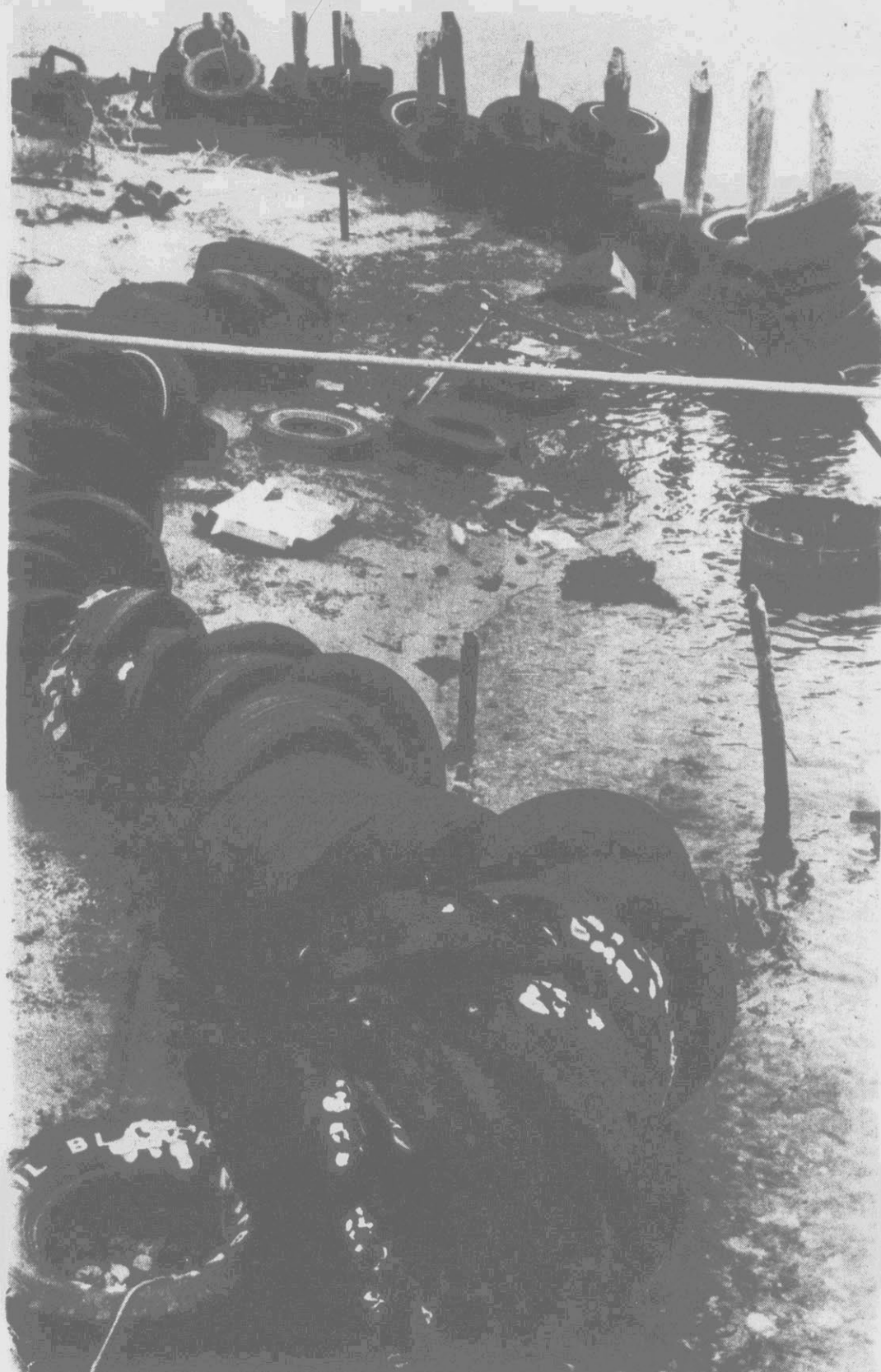
OLD RUBBER SERVES A SECOND ROLE — Worn out rubber vehicle tires are being utilized to help serve efforts to protect the environment. Along a shore in the Carteret County fishing village of Davis, tires on stakes
