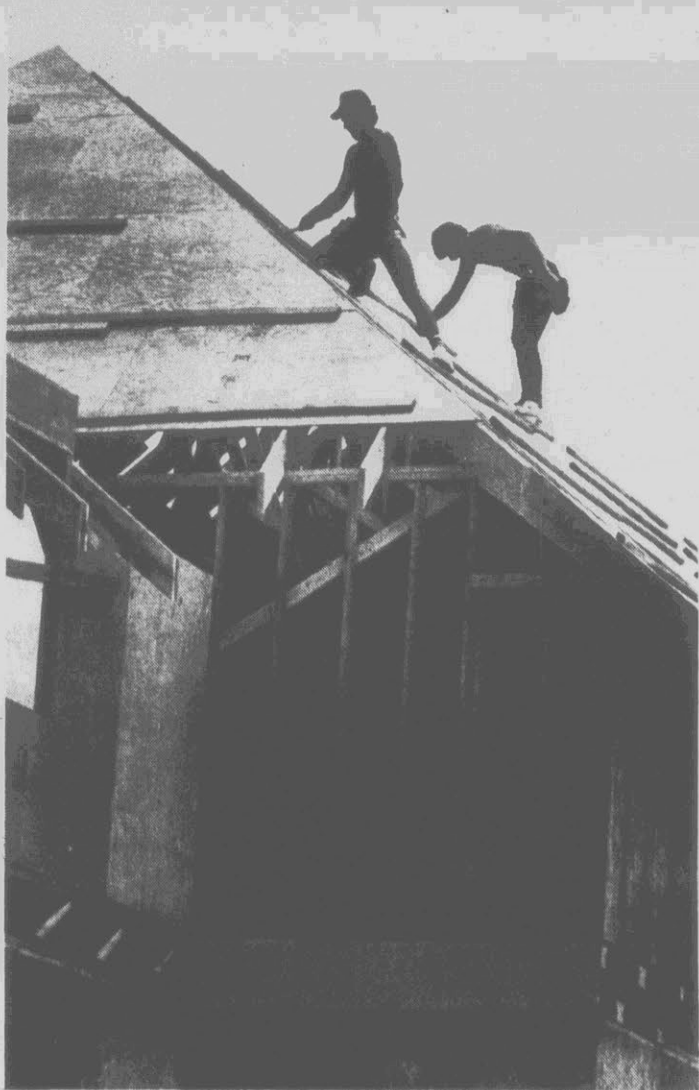
HOT TIME ON THE THIRD STORY — Construction workers Michael Rose, left, and Ken Tilley brave the hot weather as they nail part of the roof on one of the Kingston Condominiums on Greenville Boulevard yesterday. Temperatures will remain in the high 80s through the weekend with high in the 90s on Monday. (Reflector Photo by Tommy Forrest)
