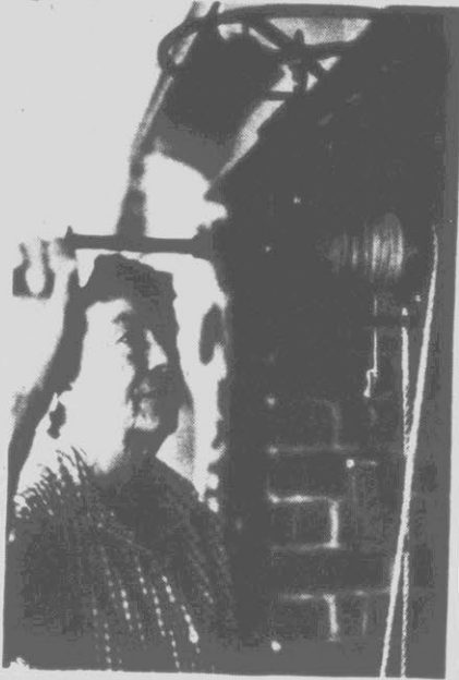
Elizabeth Midyette, New Bern, winds up the weight that in its slow fall turns the pulley and rope leading to the 200-year-old spit in front of the fireplace. It works.
