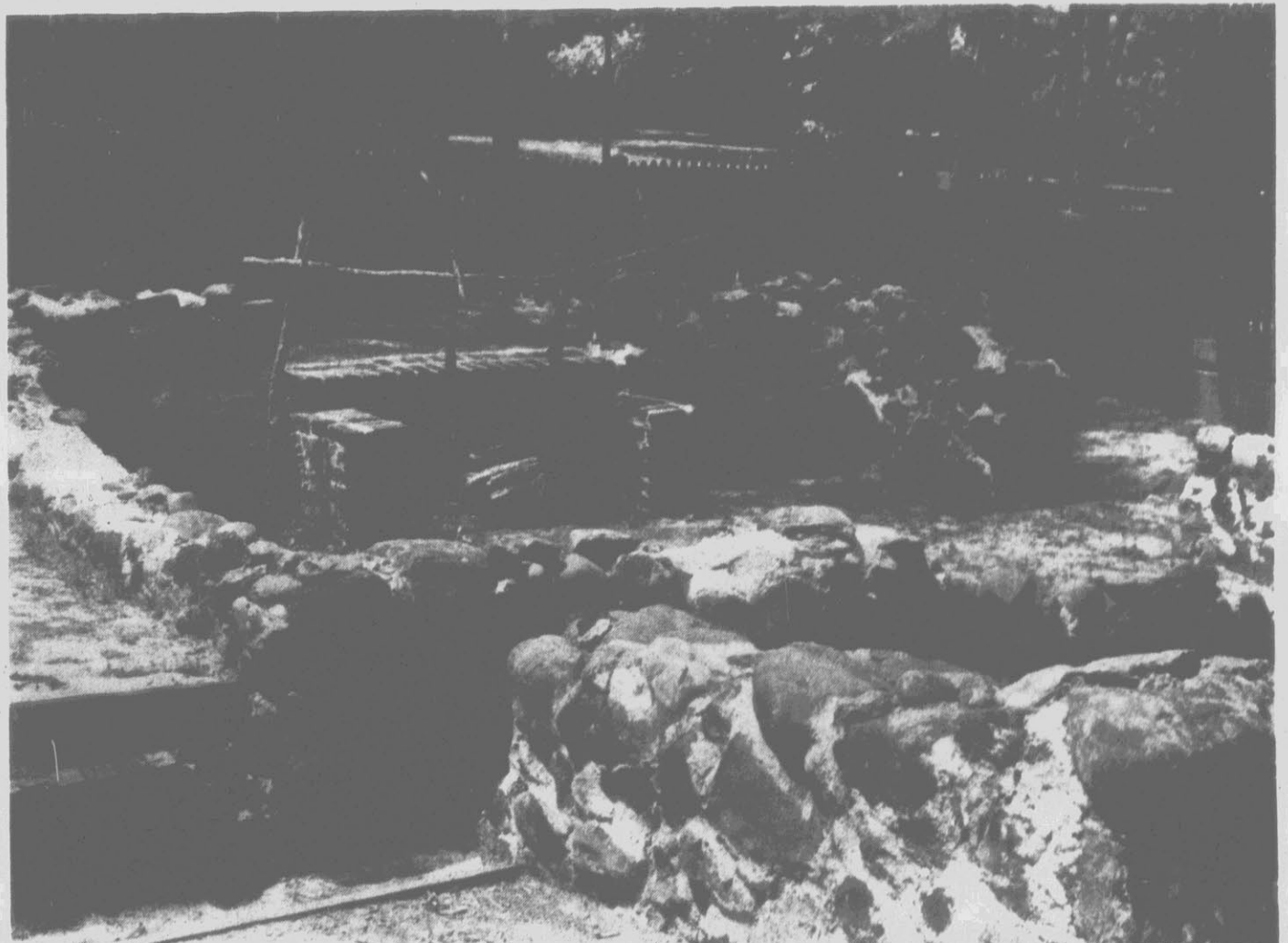
A TYPICAL FOUNDATION . . . excavated under the direction of archaeologist Dr. Lawrence Lee between 1958 and 1968 is the Hepburn-Reynolds House on Cross Street. The house is one a dozen sites where
