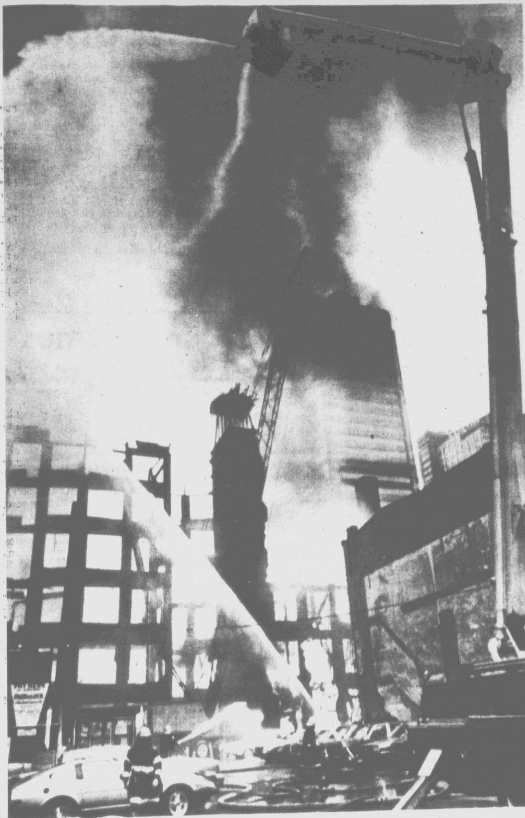
PHILADELPHIA FIRE — Firemen battle a multiple alarm fire, blamed on sparks from a torch being used by a demolition crew, in Philadelphia Thursday. The fire destroyed an eight story building, damaged at least 17 others and forced the evacuation of 25,000 people. (AP Laserphoto)
