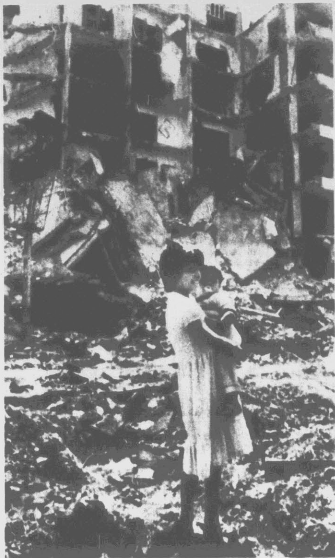
CHILDREN OF WAR — A young Lebanese girl holds her infant sister in front of what is left of an apartment building which was their home in Beirut's southern suburbs before fighting in February drove most of the civilian inhabitants from the area. Residents began returning to the area Tuesday, after a ceasefire silenced the guns along Beirut's "Green Line". (AP Laserphoto)
