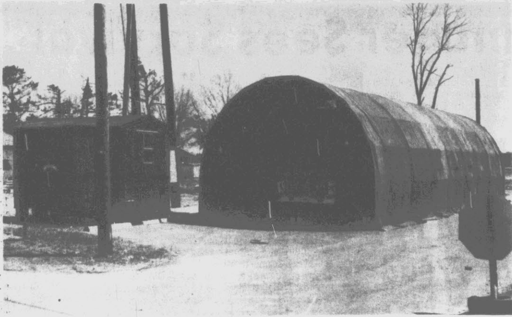
TEMPORARY SHELTER ... The Simpson Fire Department fire truck is being temporarily housed in a tent voluntarily erected by a National Guard unit out of New Bern, Assistant Fire Marshal Terry Payne said today. The department's building was destroyed by the March 28 tornado. (Reflector Photo By Tommy Forrest)
