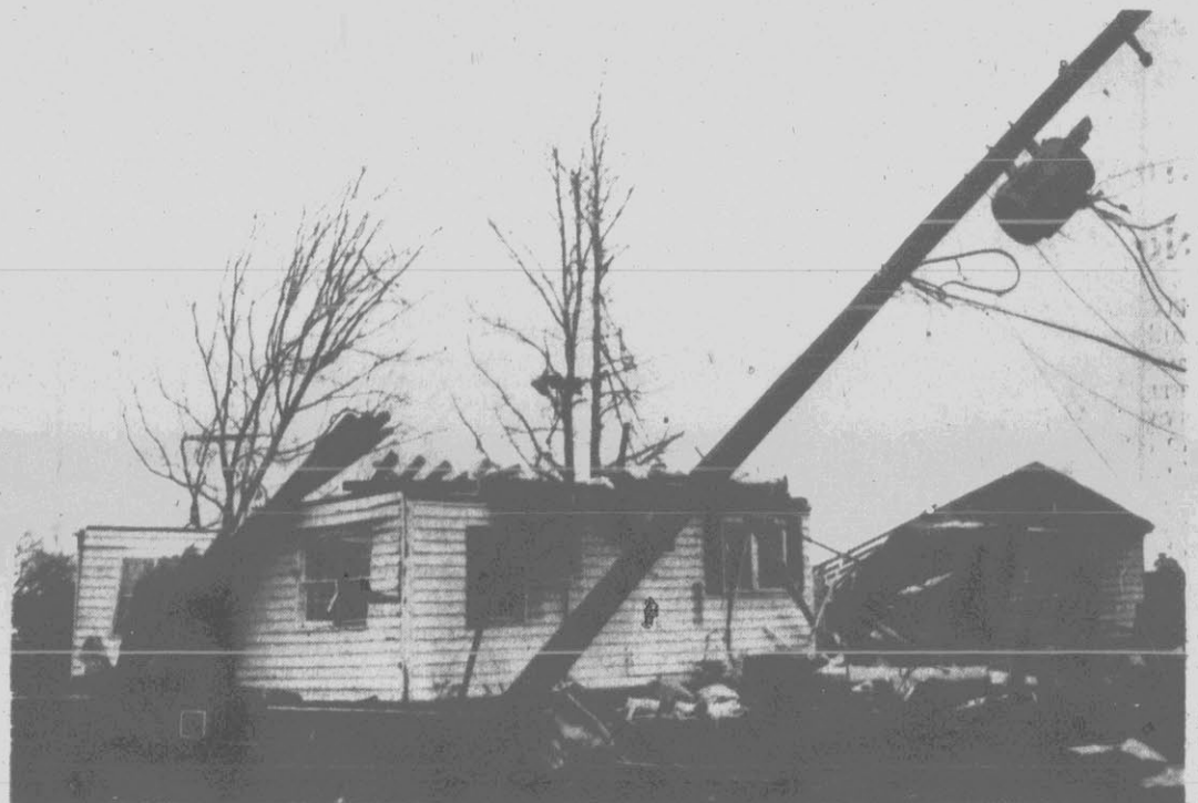
POWER LINES DOWN — Leaning, twisted utility poles and downed power lines show the random destruction left in the wake of a tornado that hit Ayden. Numerous homes and businesses were also gutted in the Ayden area during Wednesday night's storm.
