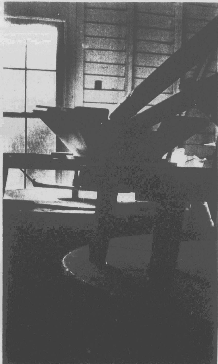
CHUTES FROM UPPER STORIES . . . feed corn into four grinding stone stations housed in circular wood structures on the ground floor.
