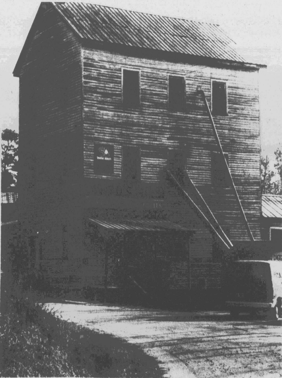
NEARLY A CENTURY OLD . . . The three story Webb's Mill, the main structure of which is shown here, was built in the late 1880s by James T. Webb. Today, the mill has a potential for
