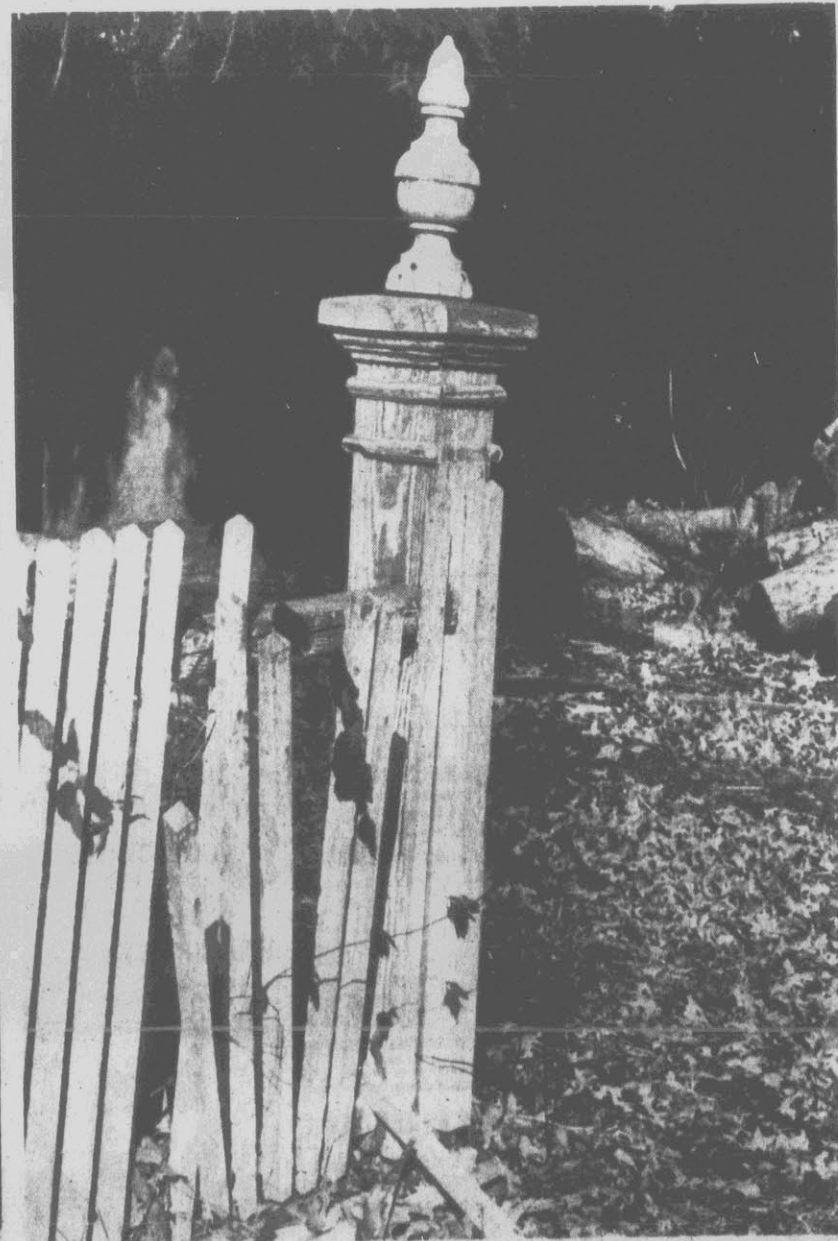
ANOTHER YEAR SURVIVED . . . A corner post and segments of a picket fence with white paint flaking away have survived the passage
