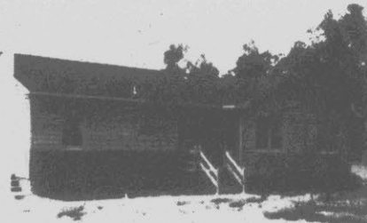
Bill Clark Construction Co., Inc. Lot #232 Beth St., Cherry Oaks
