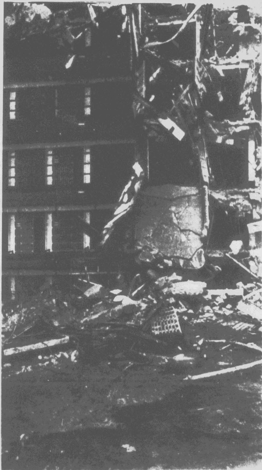
DEMOLITION — The old Central Prison, described as an imitation medieval or Gothic fortress, is being torn down in Raleigh. Workers say the demolition should be completed by November or December. (AP Laserphoto)
