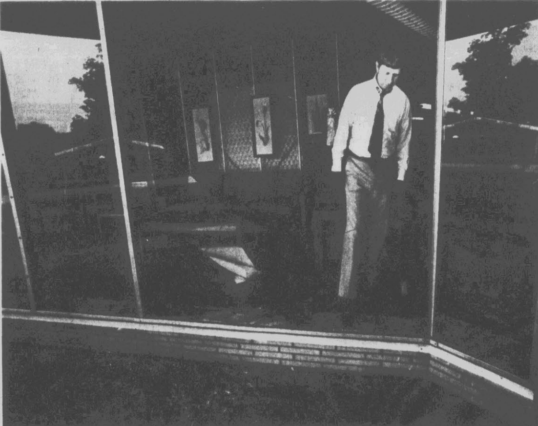
APPARENT WIND DAMAGE — Bruce Johnson of Taft Office Equipment Co. on Evans Street looks over part of a plate glass window that was
