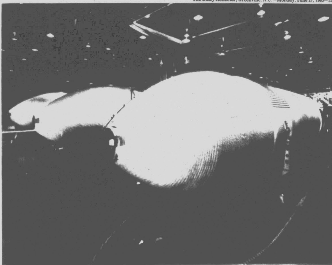
KING-SIZE FUEL TANKS — Three nearly completed Space Shuttle external tanks are lined up side by side at the National Aeronautics and Space Administration's Michoud Assembly Facility in New Orleans. These are the tanks that help boost
