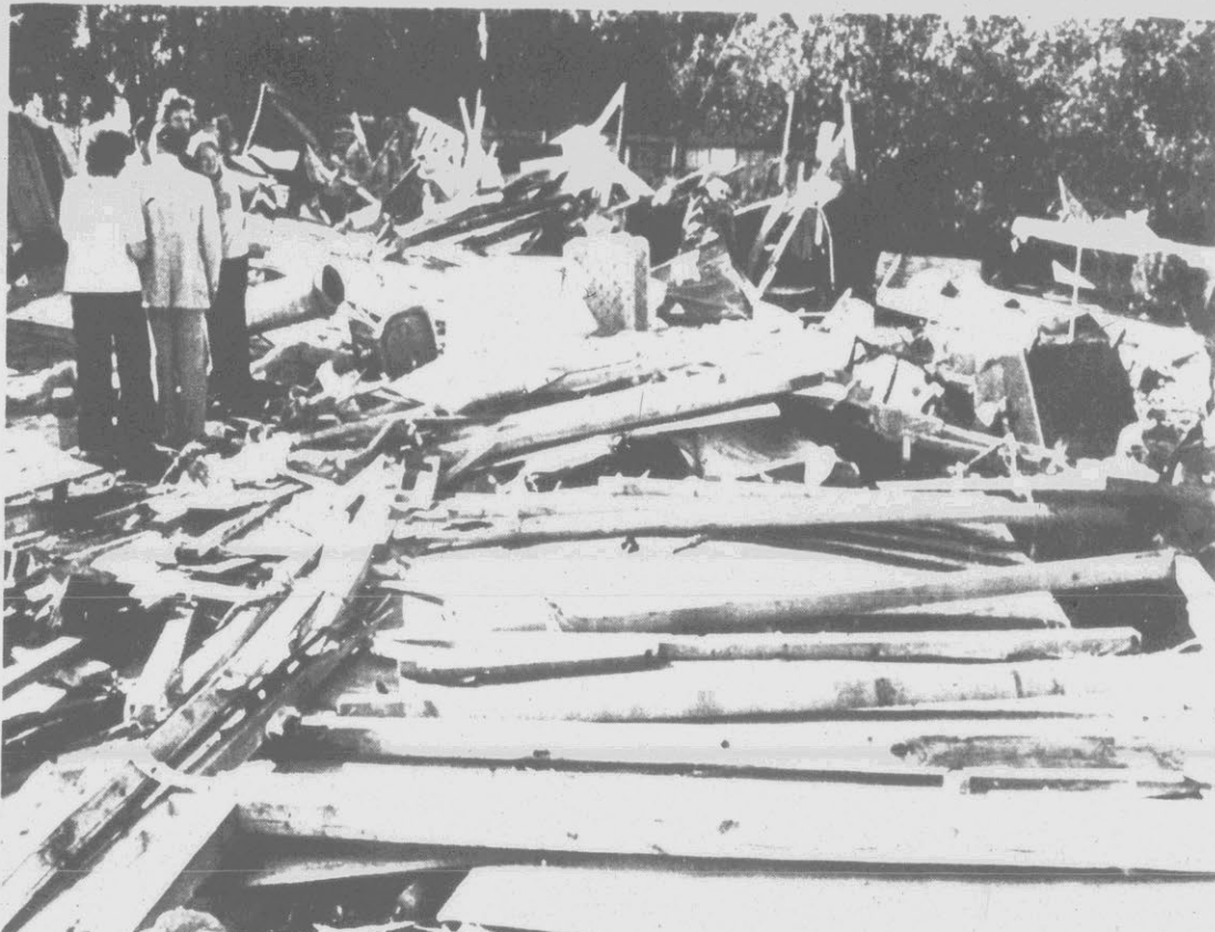
TORNADO DAMAGE — Bonnie Russell stands amid the rubble left by a tornado that struck the mobile home she was in at 4:30 p.m. yesterday. Winds moved the double-wide from its foundation
