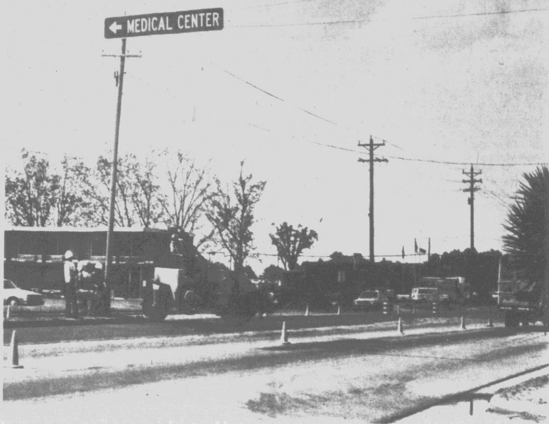
NEW TURN LANE ... Members of the State Department of Transportation work on a new double left turn lane at the intersection of Stantonsburg Road and Memorial Drive Thursday. The $15,000 lane is scheduled to be finished
