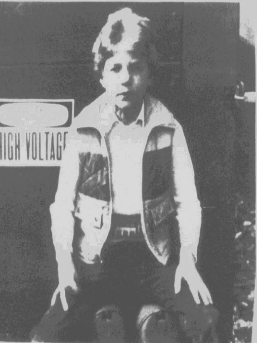
BIG SETTLEMENT — Gregory Blevins Jr., 9, of Pontiac, Mich., is shown by the transformer where he was burned on July 2, 1981. Gregory, then seven, was playing with his younger brother Robert when he opened an unlocked electrical transformer behind a shopping center. He received a shock that set his clothes on fire and caused third degree burns over 41 percent of his body. An Oakland County Mich. Circuit Court judge has signed a consent judgment calling for an initial payment of $1,052,000 and annual payments for the rest of the boy's life. If he lives to retirement age, 65, the settlement is worth $22 million. (AP Laserphoto)
