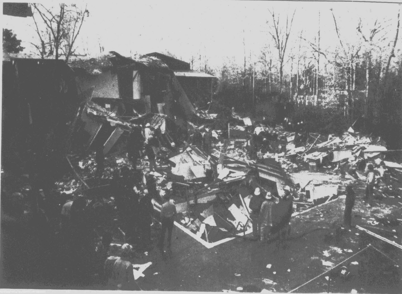
DESTRUCTION ... A view of the Village Green section of the apartment complex. (Reflector Photo by Tommy Forrest)
