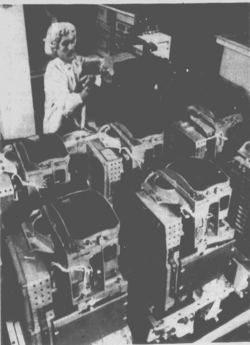
THE BETTER TO SEE 'EM WITH — Shawn Winter, a technician at Hughes Aircraft Co. in El Segundo, Calif., tests devices that enable crews of the U.S. Army's new Abrams tank to see targets at night. Hughes says the device, called a thermal imaging system, also enables the crews to see through battlefield smoke and
