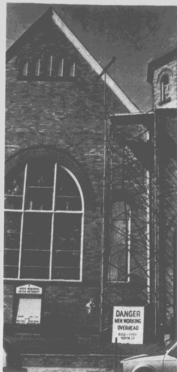
THE SIGN SAYS IT — The sign workmen placed below a scaffold leaves one thinking. In reality, there were men working overhead. Workmen have been busy over the last few weeks replacing the roof on the Jarvis Memorial United Methodist church located on Washington Street. (Reflector Photo by Tommy Forrest)
