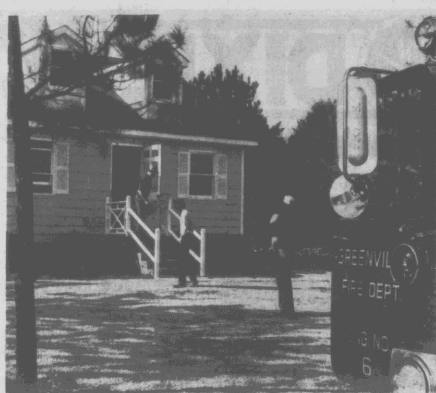
HOUSE DAMAGED IN TUESDAY FIRE — Greenville fire-rescue personnel clear smoke from a residence at 104 Osceola Drive shortly before noon Tuesday. According to department records, the owners of the house were listed as William Faulkner and George Dunn. The fire, which was confined to the den of the
