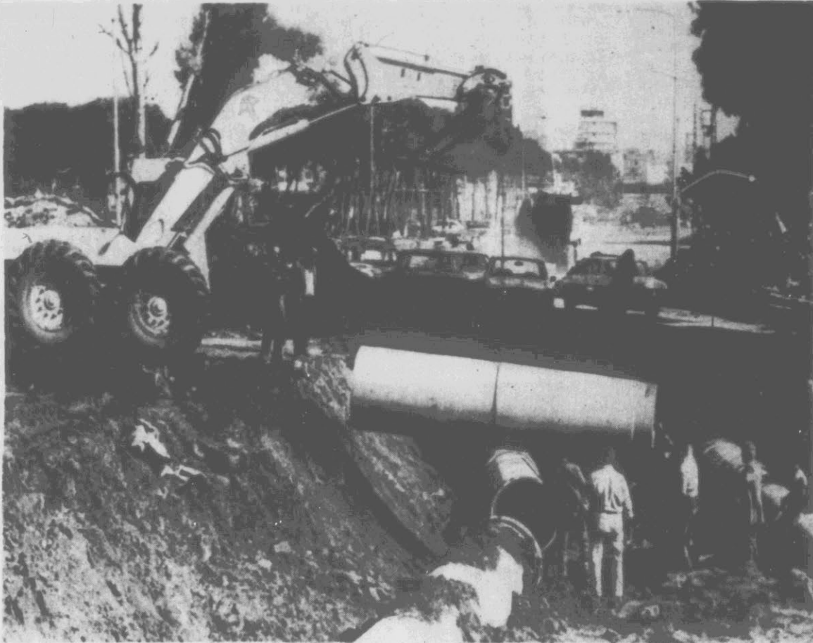
REPLACING PIPES — Workmen replace pipes in West Beirut as the streets echo with the sound of hammering and grinding of cement mixers.
