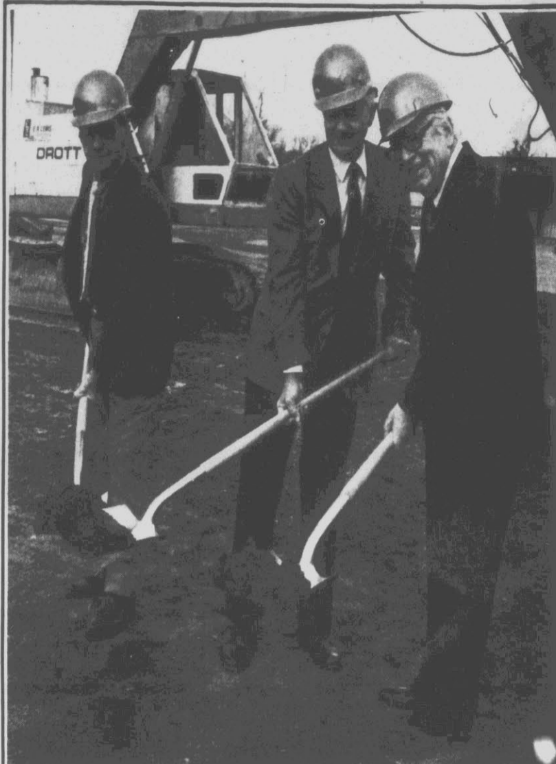
TRANSIT GARAGE GROUND BROKEN ... Officials breaking ground this morning for the new transit garage were (left to right) J. H. Hudson, general contractor, Mayor Percy Cox, and former City Councilman Frank Fuller, chairman of the Public Transportation Commission. (Reflector Photo by Tommy Forrest)
