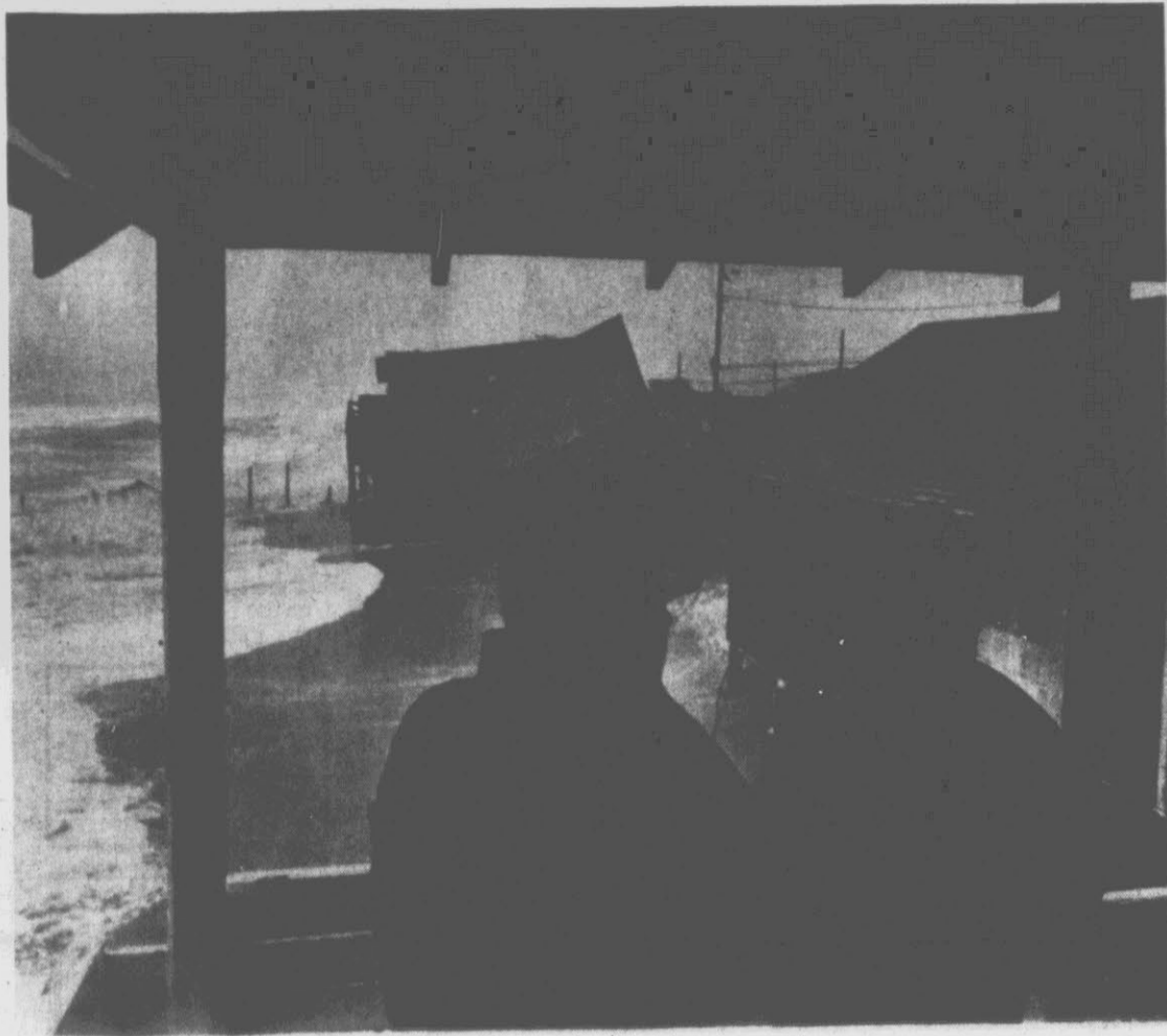
SURVEYING THE DAMAGE - High winds and stormy seas destroyed this house and blew the side of another at Kitty Hawk this weekend. (AP Laserphoto)
