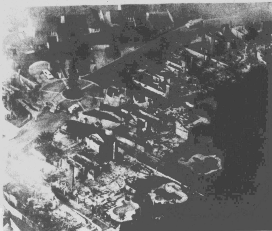
SUBDIVISION DEVASTATED — An aerial view shows the destruction at Crest De Ville subdivision in the city of Orange, Calif., after a Gypsum Canyon fire burned 18,000 acres and destroyed 56 houses in the area southeast of downtown Los Angeles. (AP Laserphoto)
