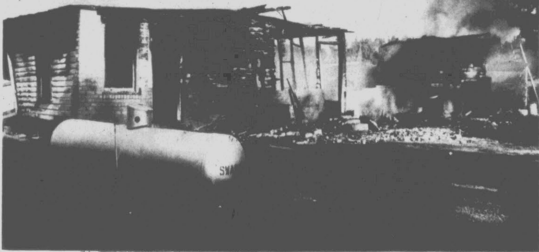
CLUB DESTROYED BY FLAMES — "The Hideout" club located near Grimesland off rural paved road 1760, was destroyed by fire early Sunday morning. According to the owner Elmond Hardy, the club had not been occupied since Saturday night, a week ago. The owner said he was asleep in his house, which is located next to the club, when the fire was
