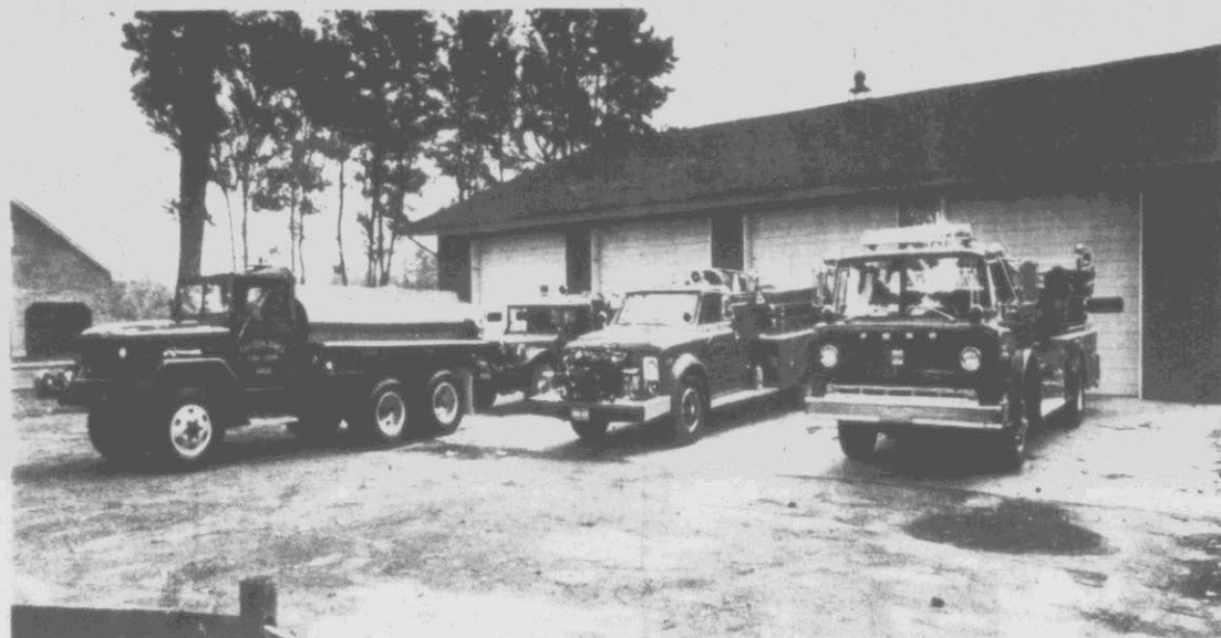
Eastern Pines Firefighting Equipment At Ready
