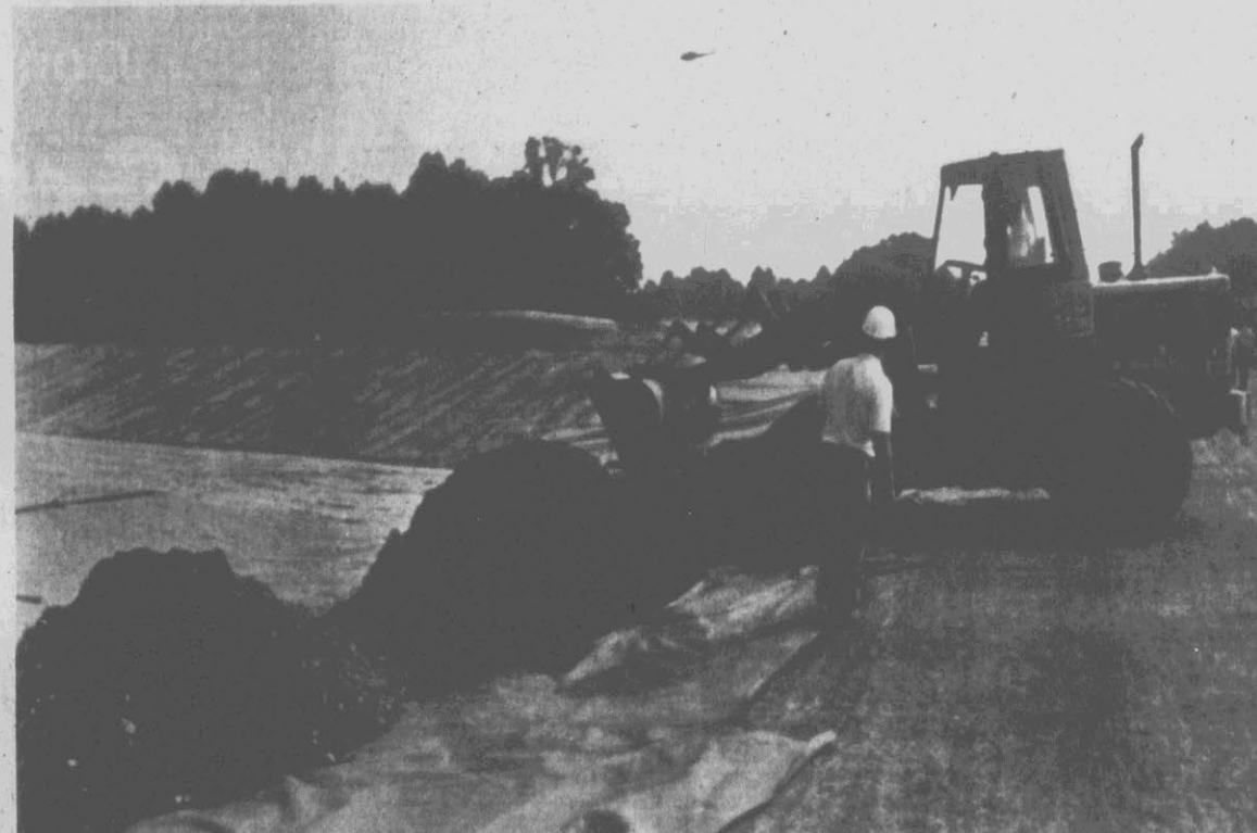
CONTROVERSIAL LANDFILL — Workers dump soil containing a toxic chemical being scraped up from North Carolina roadsides as a
