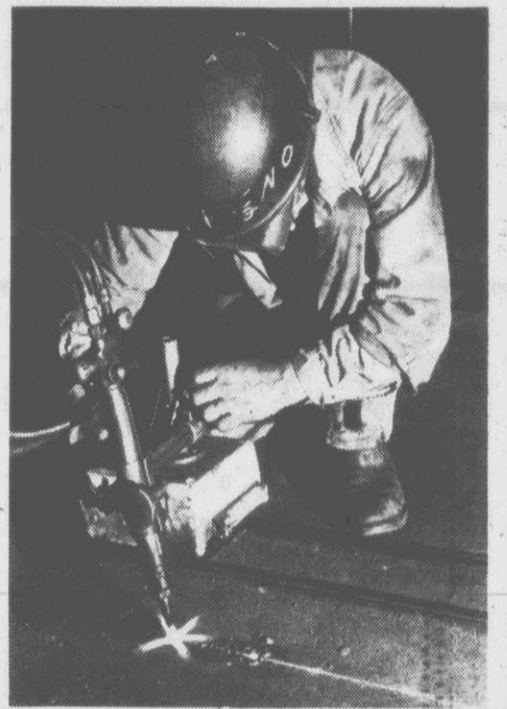
Cutting line, just forward of bridge.
